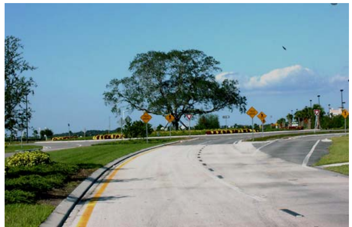
Figure 13 A new two lane roundabout in Viera, Florida. Note the size of tree that was moved to create the centerpiece.
