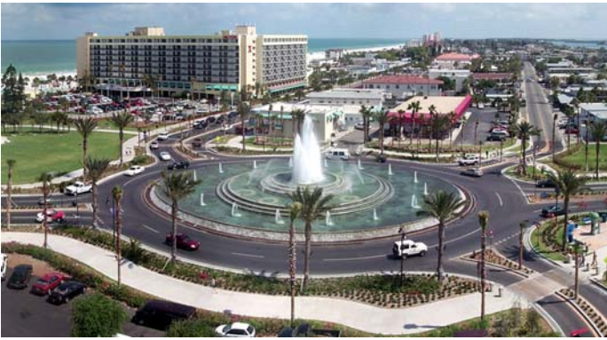
Figure 9 An overview of the Clearwater Beach Roundabout
