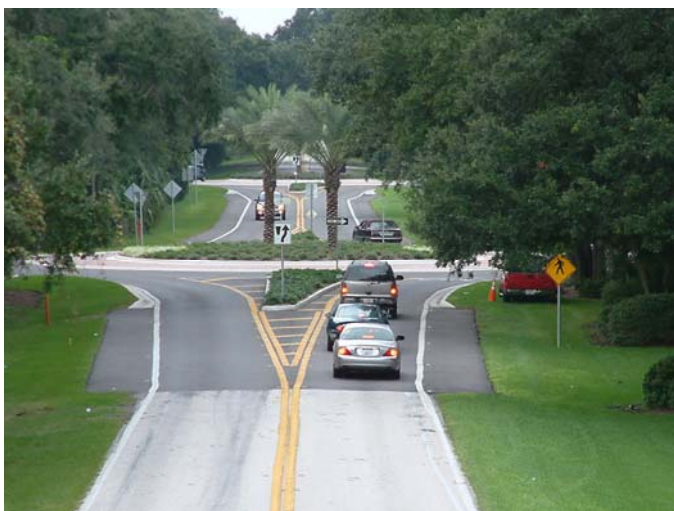
Figure 11 Twin roundabout only 600 feet apart on A1A in north Florida in a 45/55 mph zone.
