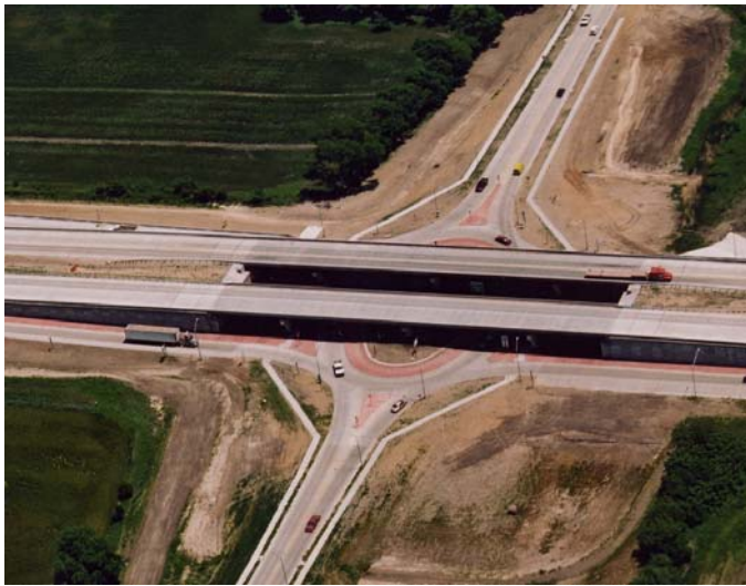
Figure 10 Tight Freeway Interchange in Newton , KS
