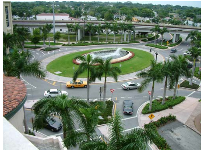
Figure 12 Cover Photograph A beautiful roundabout at the entrance to an upscale shopping mall in Coral Gables. Roundabout is located on a four lane road at a six leg intersection carrying approximately 2,000 vehicles per hour.
