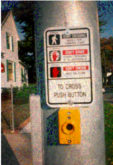
Figure 1. An illuminated push button in Windsor. The orange light is below the button.
