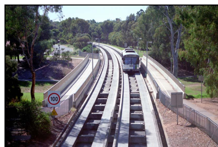
(b) Guided Busway (Adelaide, Australia)
