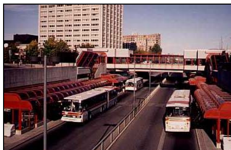
(a) Grade-Separated Busway (Ottawa)
