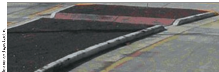
Figure 3. Barrier curb on the splitter island.
