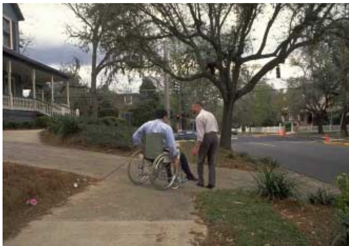
Driveway slopes should not encroach into the sidewalk.
