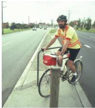
This median provides a diagonal waiting area for bicyclists, including a railing to hold onto.
