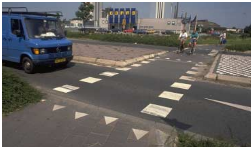
These pavement markings at a median refuge not only delineate the crossing for motorists, but also cue pedestrians about the location of the roadway edge.
