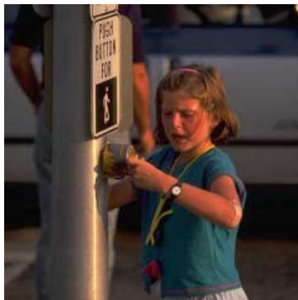
Pedestrian push buttons are often provided at locations with intermittent pedestrian volumes to call for the WALK message and/or extend the crossing interval.
