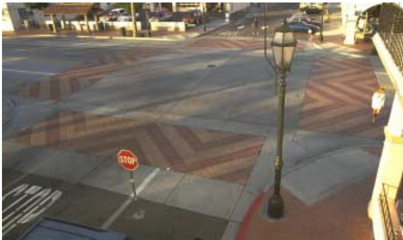
Pavement treatments can be applied to the entire traffic-calmed area or limited to specific street uses. The texture or color should be a noticeable contrast to the approaching roadways if speeds are to be reduced.
