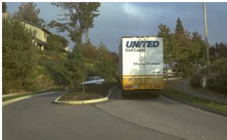
This traffic-calming measure uses a landscaped median to narrow the travel lanes.
