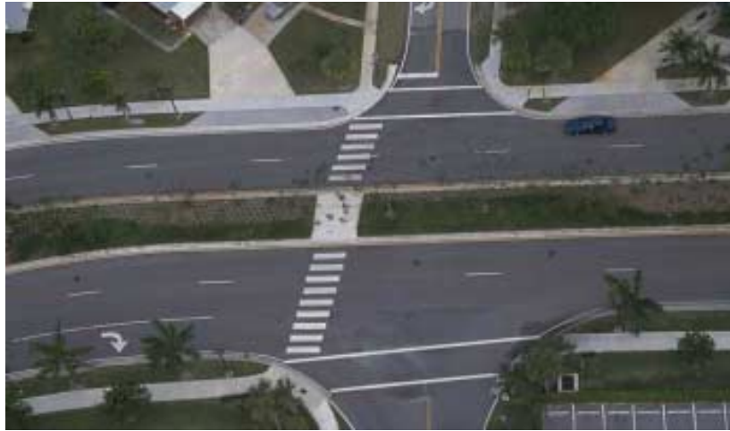
Refuge islands provide pedestrians with a resting place when crossing roads or intersections.
