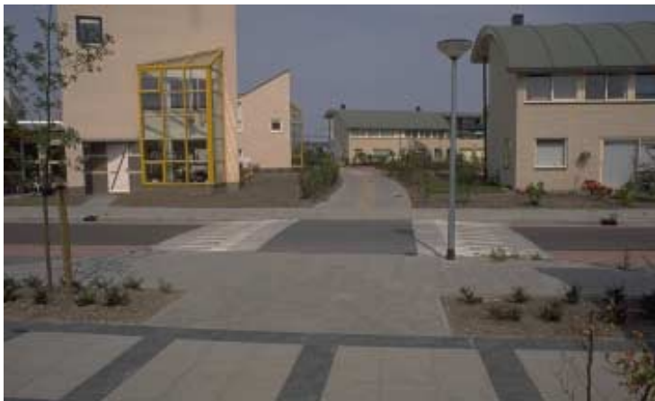
Raised crosswalks can both slow motor traffic and give pedestrians a continuous-level surface at the crossing. Changes in texture and color help define the edges of the crossing.
