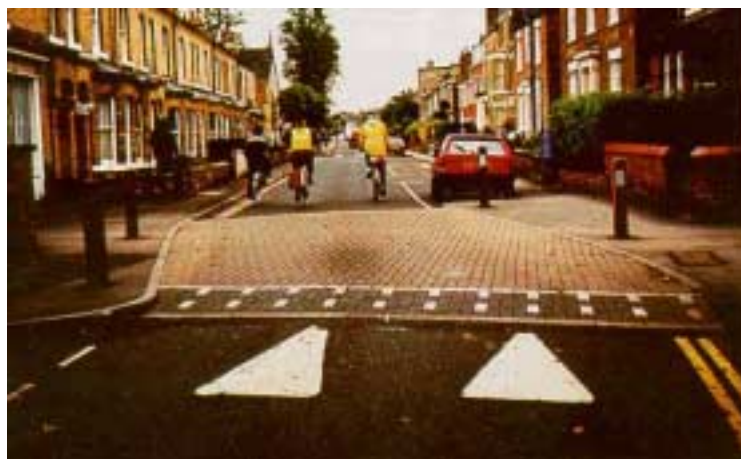
Speed humps slow traffic speeds on residential streets.
