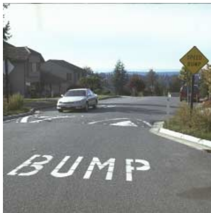
Speed bumps can be combined with curb extensions and a winding street alignment. Signing and pavement markings should clearly identify the bump.
