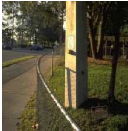
This pedestrian signal would not be accessible to all users. How can a child reach this to cross the street safely?
