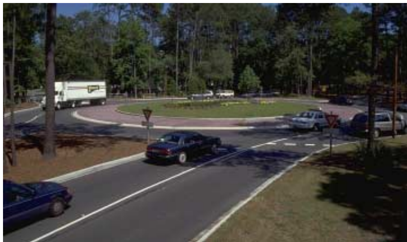
Traffic circles can be designed to accommodate large vehicles and emergency access without undue restrictions.
