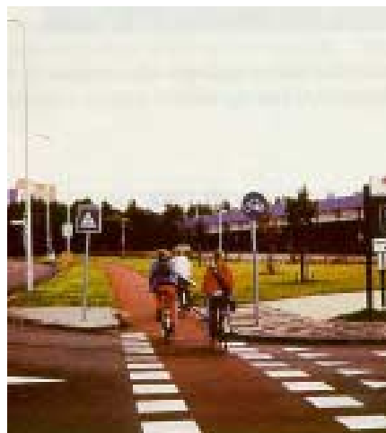
FIGURE 23-8. Some bicycle paths parallel roadways, such as this one in Groningen, The Netherlands.
