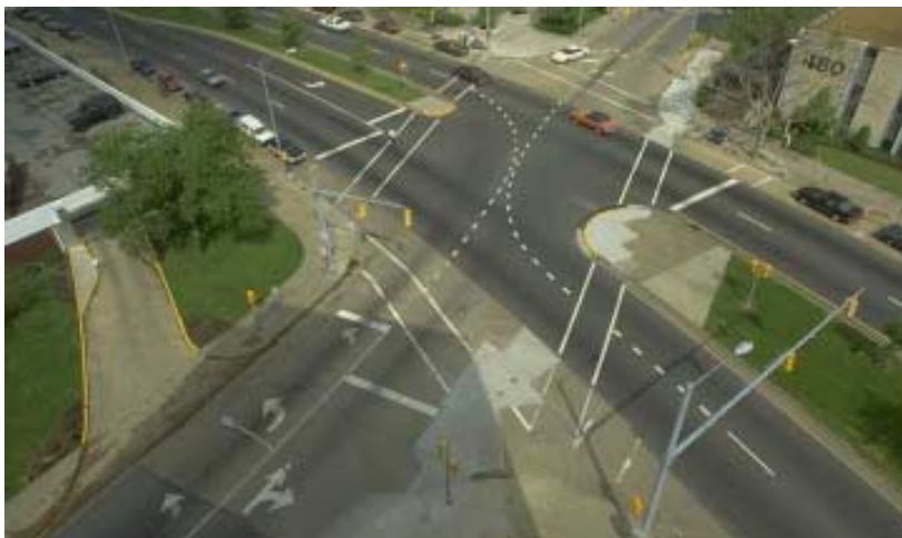
Pedestrian refuge islands can create a safer crossing for wide streets.
