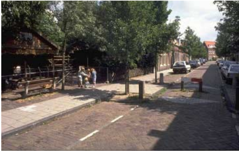
The design of street closures should provide specific parking areas to discourage obstruction of bicycle and pedestrian traffic.
