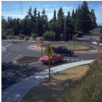
The splitter islands should be raised and landscaped to prevent left-turning vehicles from taking a short cut to avoid driving around the outside of the island.
