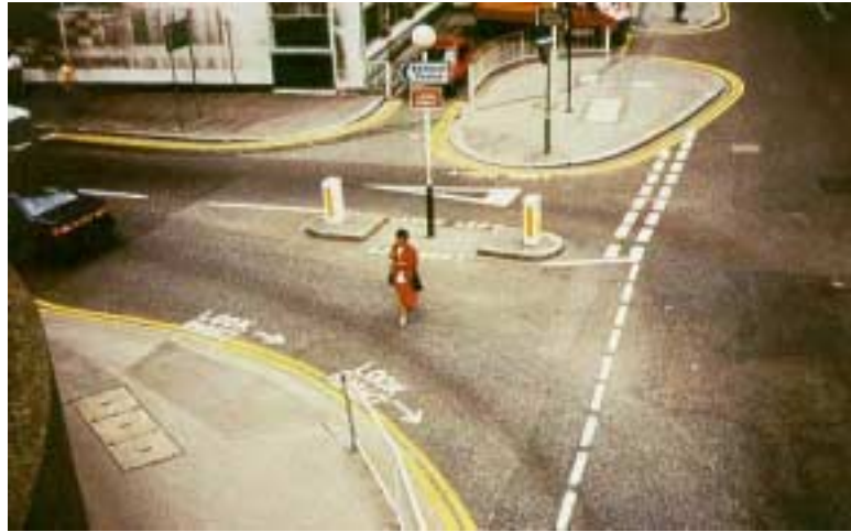
FIGURE 23-5. Pedestrian pavement messages and refuge islands.
