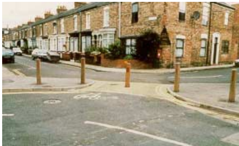
Diagonal road closures/diverters limit vehicular access, but allow emergency vehicles to enter through removable bollards.
