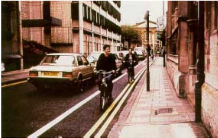
Figure 23-15. Contra-flow bicycle lane in Cambridge, England.
