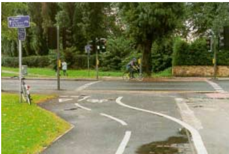
Figure 23-4. Toucan crossings in Great Britain provide separate pedestrian and bicyclist signals where trails cross roadways.
