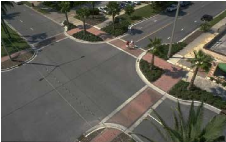
Traffic calming can be termed as engineering and other physical measures designed to control traffic speeds and encourage driving behavior appropriate to the
