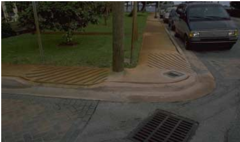
A 7-foot radius allows for a slow and safe turn. As the radius increases, so does the speed of the vehicle.
