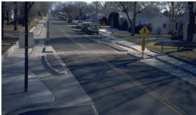
Where possible, cyclists should be provided with cycle slips which enable them to bypass speed humps.
