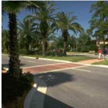
Midblock crossings are easily located on low-volume, low-speed roadways, such as short collectors through neighborhoods.
