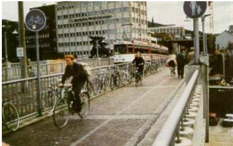
A pedestrian and bicycle bridge near the Freiburg rail station carries thousands of people each day.
