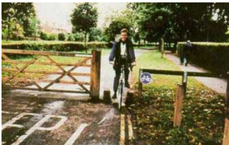
Figure 23-17. Entrance to bicycle trail is designed to restrict entry by motor vehicles.
