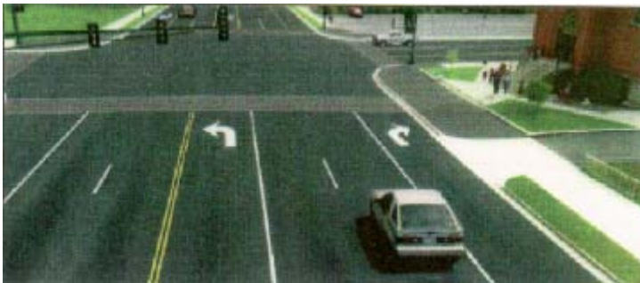
Example of dedicated turn lanes with separate lanes for “through traffic.” Federal Highway Administration, Flexibility in Highway Design chap. 6 (1999).
