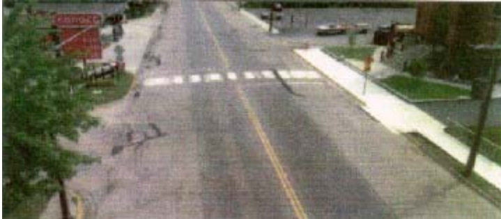
Street without dedicated turn lanes and medians. Federal Highway Administration, Flexibility in Highway Design chap. 6 (1999).
