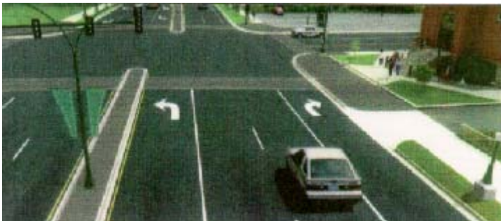
Street with dedicated turn lanes, turn lanes, median, and sidewalk buffer. Federal Highway Administration, Flexibility in Highway Design chap. 6 (1999).
