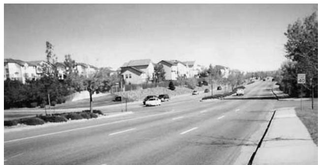
Figure 17. Conventional median opening at four-leg intersection.
